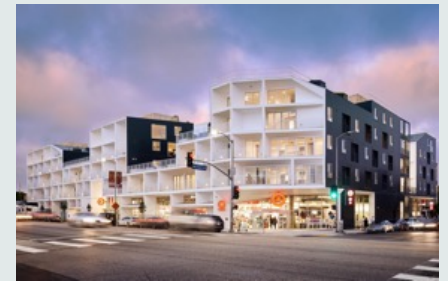
Santa Monica Westgate | Los Angeles 143,000 SF Residential, Ground Floor Retail
