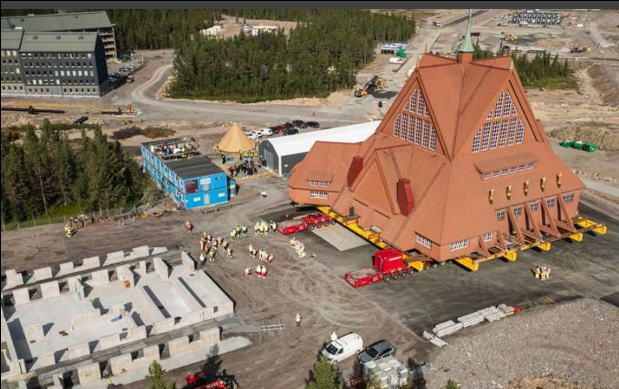
Enerpac EVO Synchronous Lifting System utilized to raise and help relocate the Kiruna Church in Sweden.
