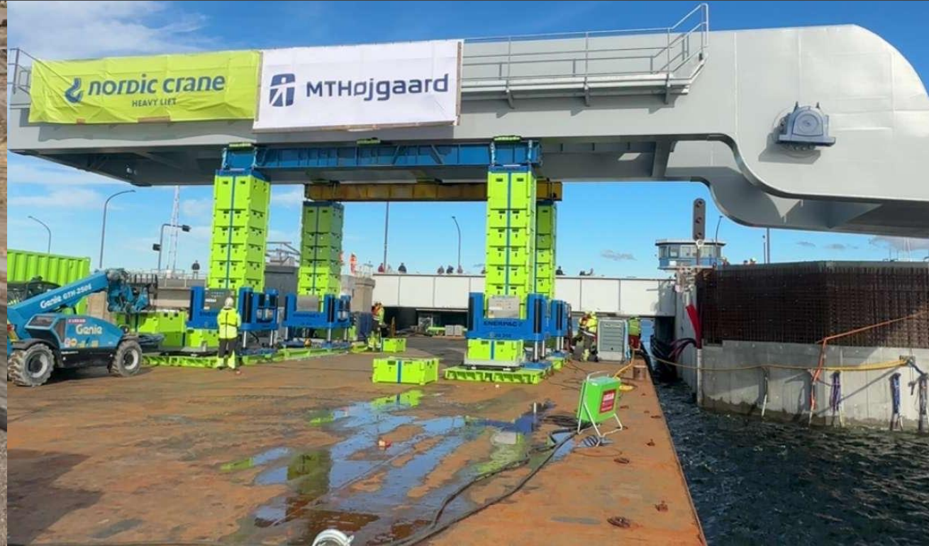
Enerpac JS250 Jack-Up System lifted and positioned 100+ ton bridge element in Denmark.
