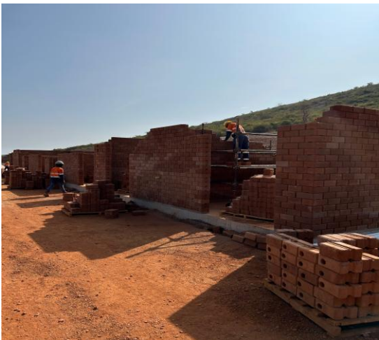
Terrace5 building Hydroform brick works Terrace 4 buildings 5, 4, 3, and 2 works
