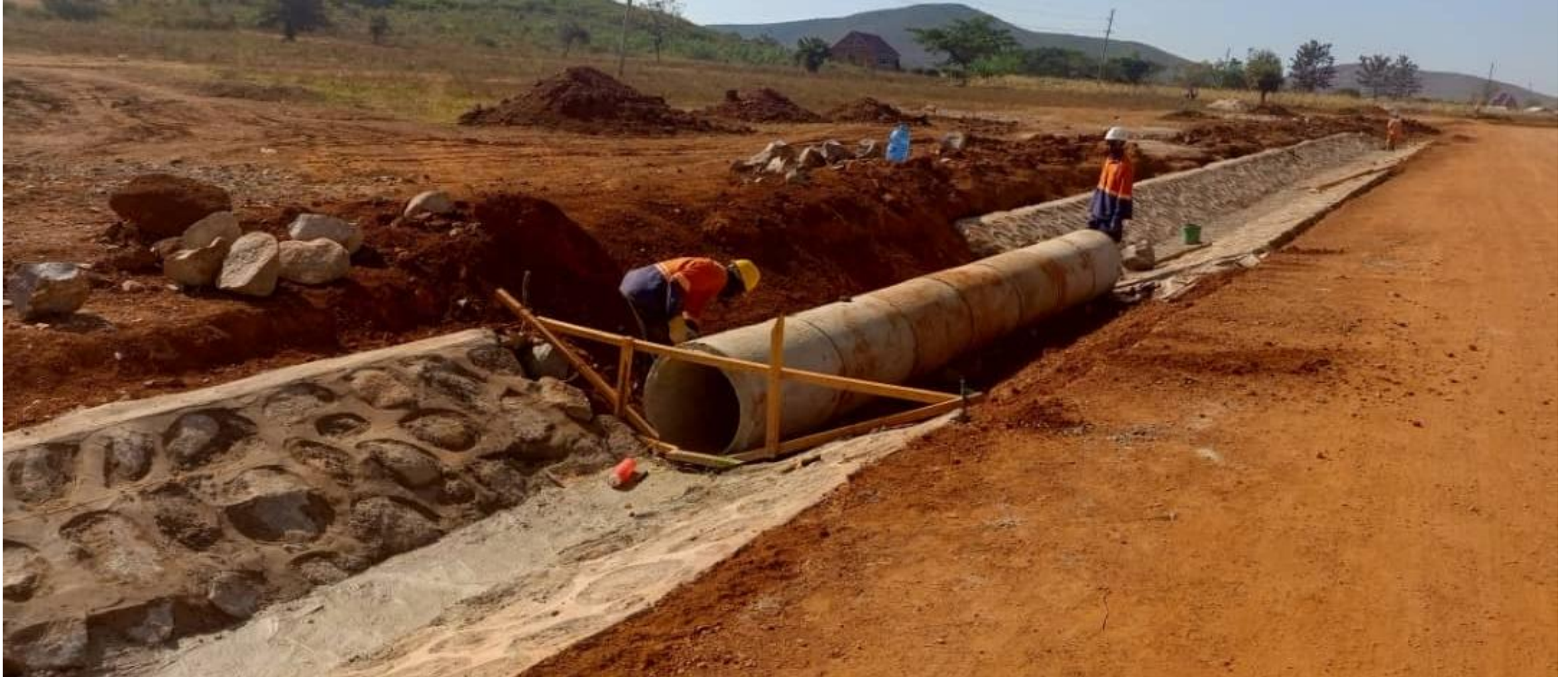
Ngoma Bypass Road – Access Road Crossing Culvert Installation.
