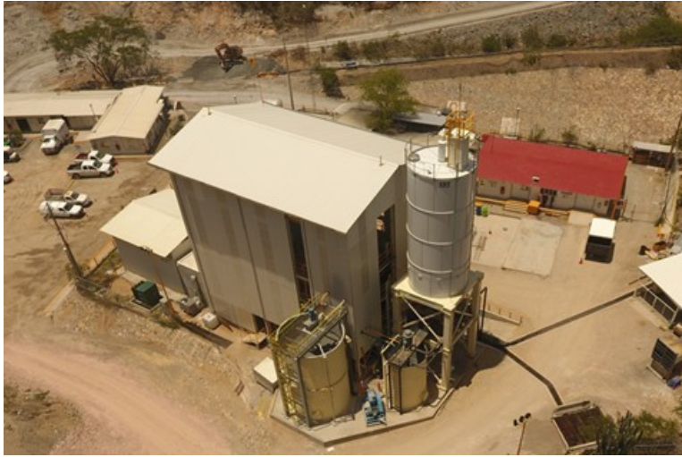
Figure 14-8: DDGM's Paste Plant.
