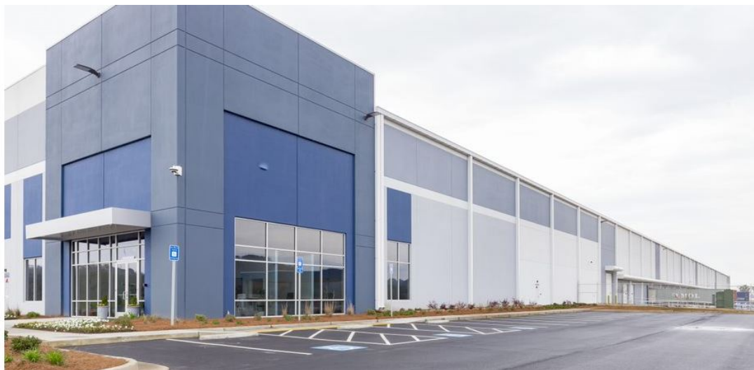
Industrial building owned by Gladstone Commercial, located in Crandall, Georgia
