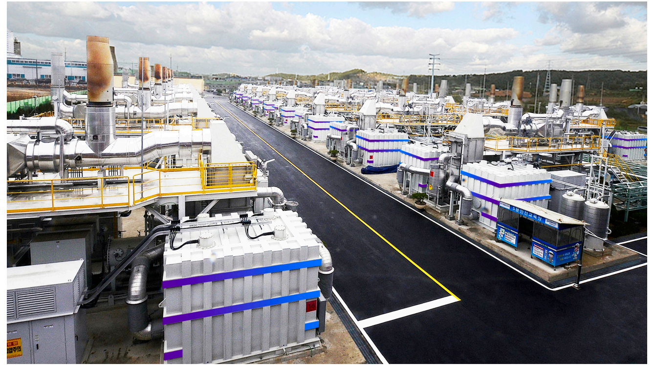
Gyeonggi Green Energy - 58.8 MW fuel cell park provides power and heat to local homes.
